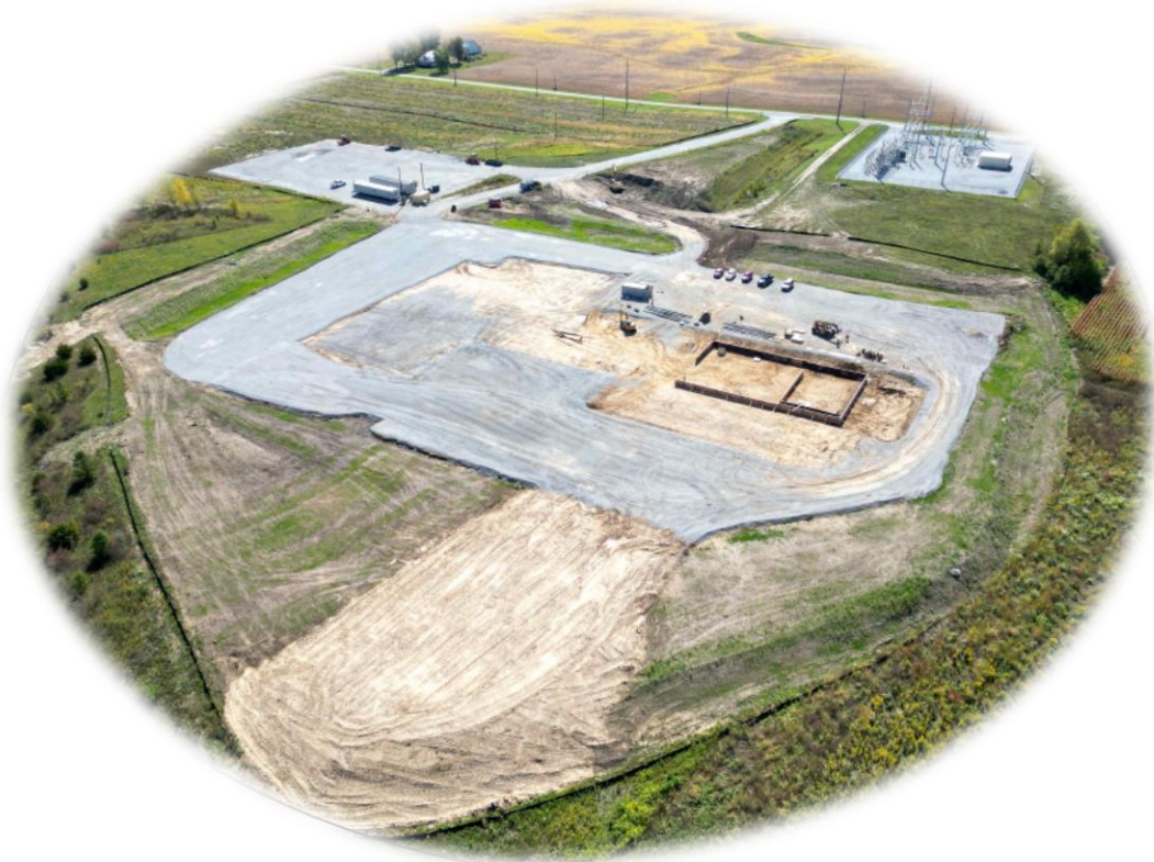
November 2023 - Concrete Foundations
