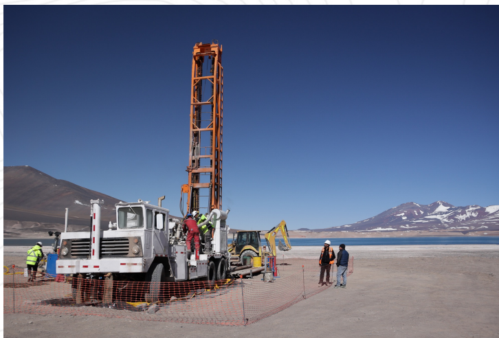
Rig mobilising at Laguna Verde January 2023
